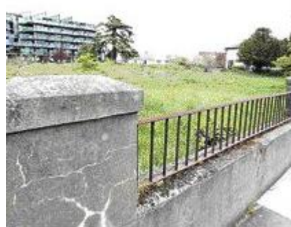
CREDIT: Bruce Stotesbury, Times Colonist A current view of the property looking on to the Reef condo complex.
